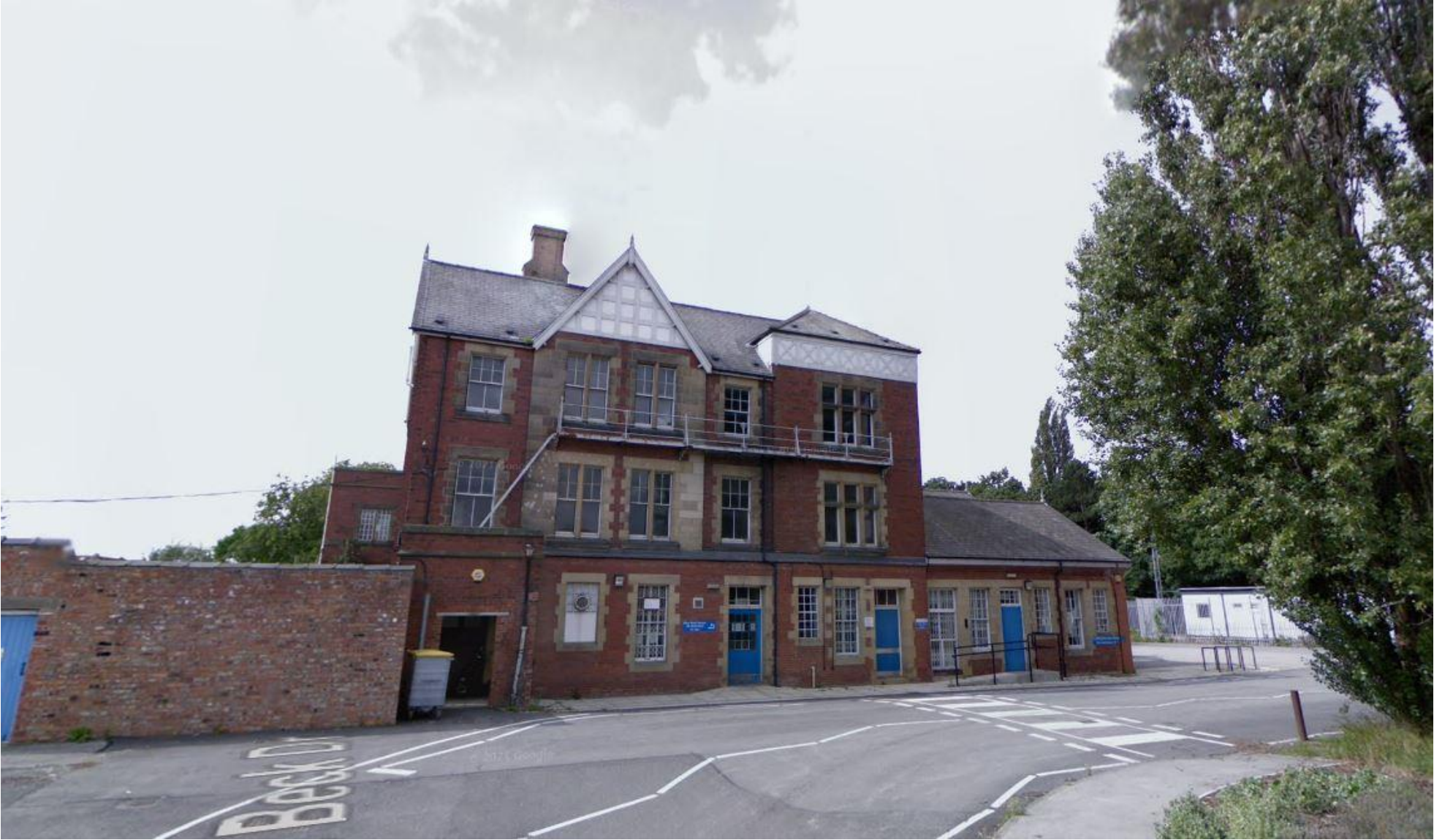
Existing Building - Front
